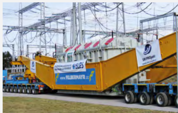
Replacement of a transformer in Divača
