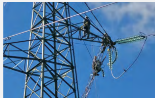
Rehabilitation of damage cause by vandalism
